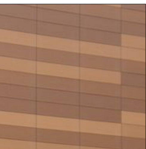
MATERIAL 4 Alucobond panels, Wood design colour 'Royal Cedar'
